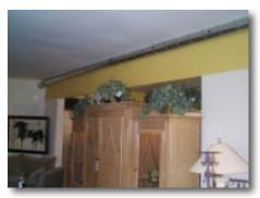
The pictures demonstrate a "drilled outlet" installation for cooling, installed by Matt Getz of Climate Control and purchased through Southern Cal A/C Supply in EL Cajon, CA. Drilled outlets are unobtrusive and have been designed to fit in and match the space they are installed into, creating a much more visually appealing effect than other possible applications.
