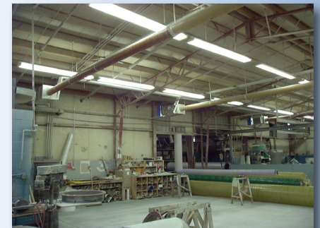
10 Hi-Velocity Fan Coils Provide Heating and Cooling
