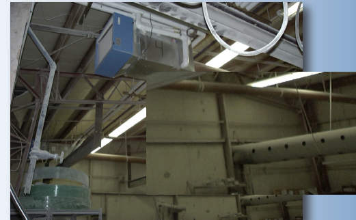
2" Drilled Outlets provide longer Air Throws
