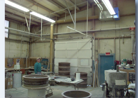
Drilled Outlets provide Shipping Door Air Curtain
