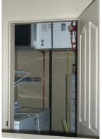
Suspend the fancoil from the ceiling above the water tank all of which shares a closet with the washer/dryer units.
