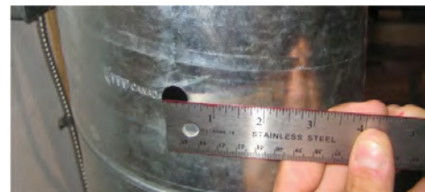
Fig. 05 - Drill 3/4" (13mm) hole
