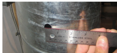
Fig. 05 - Drill 3/4" (13mm) hole
